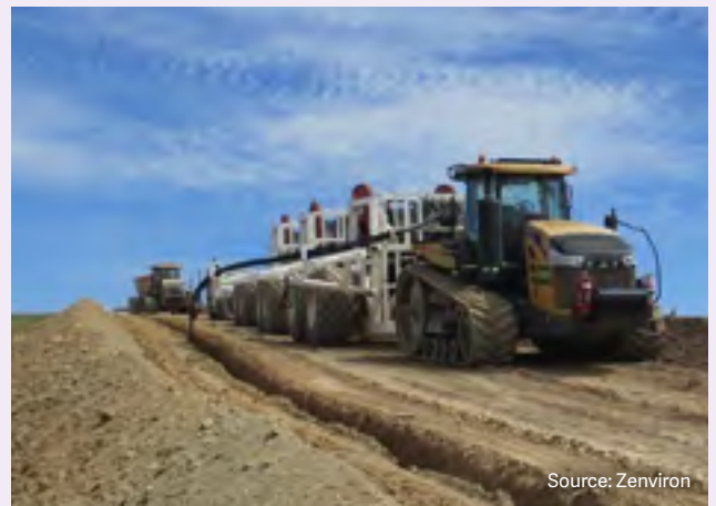
Underground or overhead electrical and fibre optic cables are installed to connect the wind turbines and carry electricity and control data to the substation.
