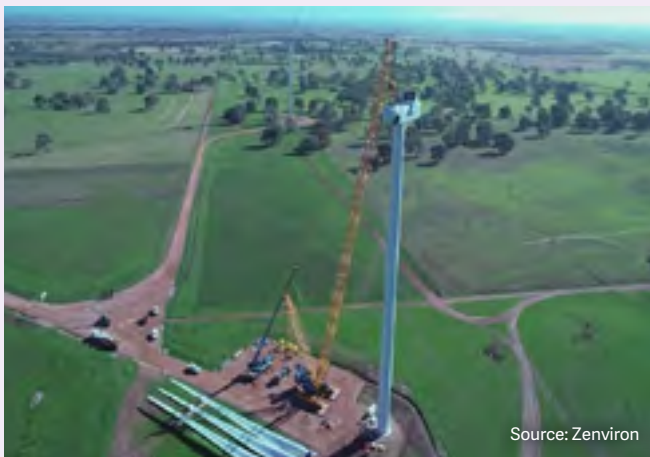
A crane uses the hardstand area to install a nacelle and rotor on top of the tower sections with the blades ready to be installed.
