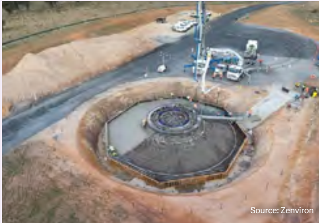
Concrete being poured at a turbine foundation
